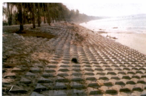
Erosion Prevention Dike in Ham Tien, Viet Nam
